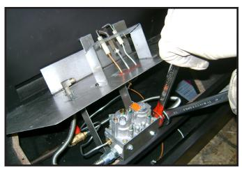
Figure 16.7 Disconnect Gas Valve
